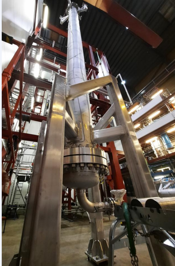
Hoisting the WGS reactor into place Positioning of SEWGS reactor 1
