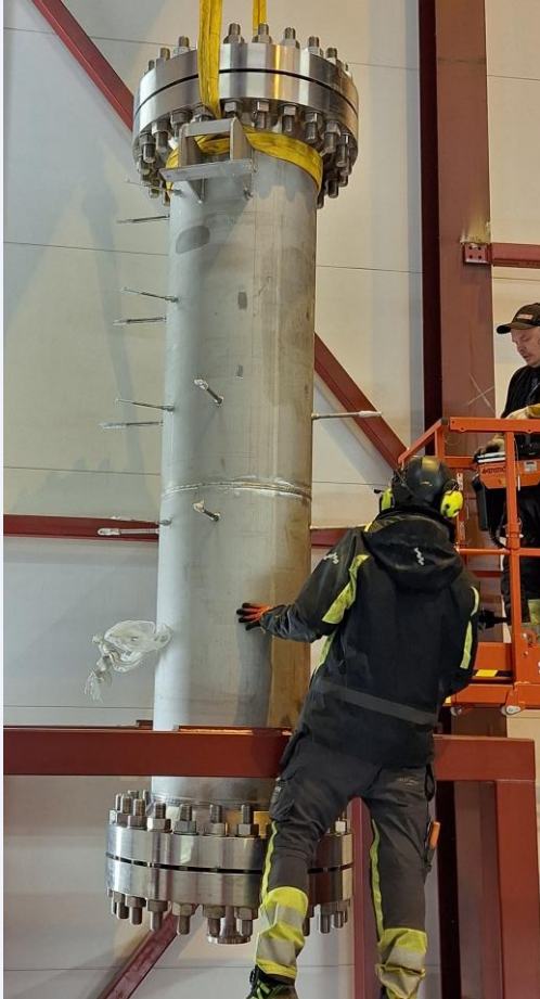
Hoisting the WGS reactor into place Positioning of SEWGS reactor 1
