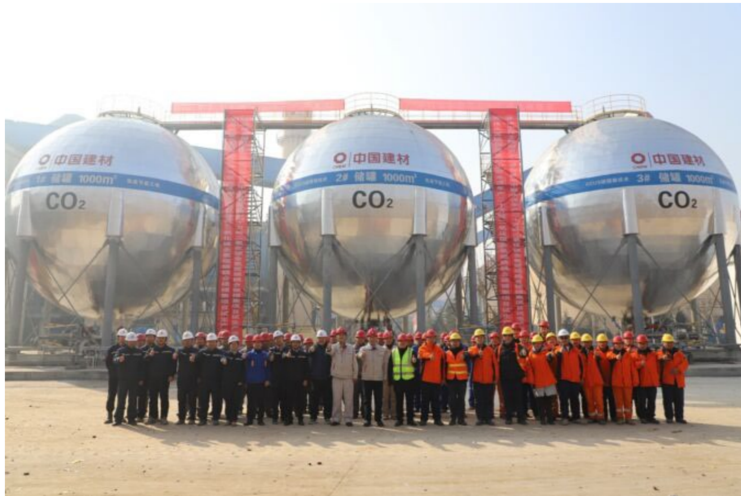
The CO 2 Storage Tanks at the Qingzhou Oxy-fuel Combustion Cement Project Site (provided by Tianjin Cement Industry Design & Research Institute)
