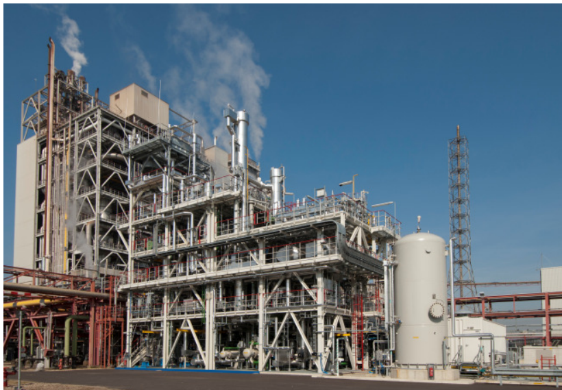
Figure 2-2: CO 2 capture pilot plant. The tall column in the middle of the picture is the CO 2 absorber.
