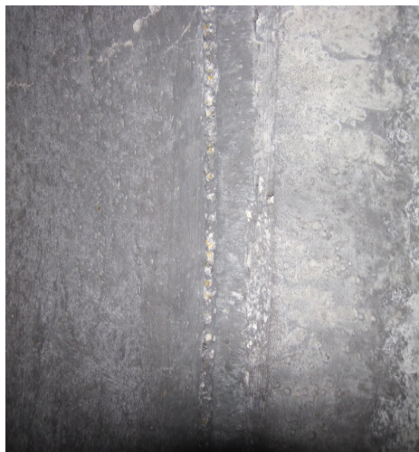
weld pipe/ pipe-cap
