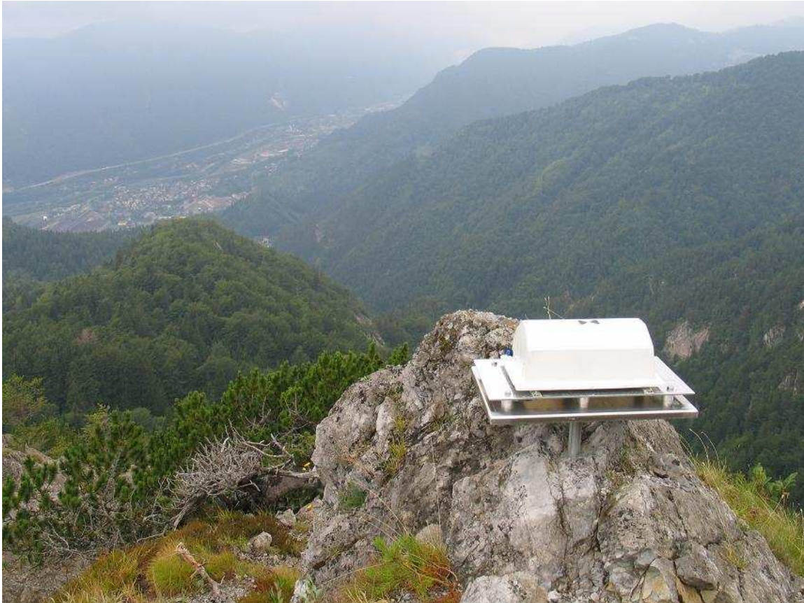
Figure 16. An installed I2GPS unit in a landslide risk area for deformation monitoring (image courtesy of GeoZS).
