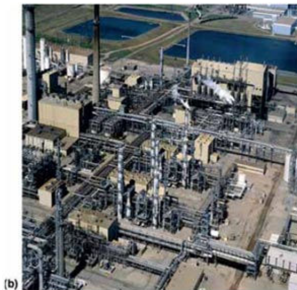
Figure 21a: This plant employs a chemical absorption process to separate 0.2 MtCO 2 per year from the flue gas stream of a gas-fired power plant for urea production (Malaysia, Courtesy of Mitsubishi Heavy Industries). (b) CO 2 precombustion capture at a coal gasification plant in North Dakota, USA. This plant employs a physical solvent
