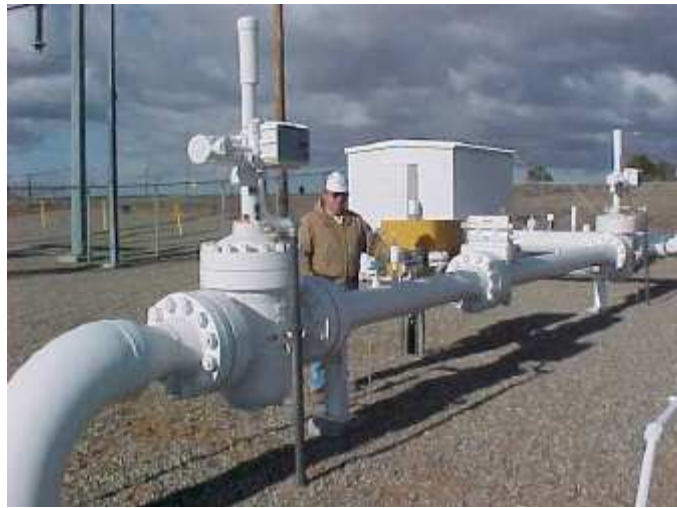
Figure 6: Inspection of the Cortez pipeline, New Mexico, U.S.A (KinderMorgan, 2006)
