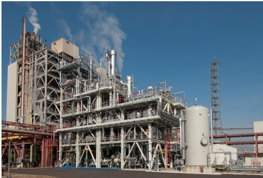
Fig. 2. Photo of the pilot plant at the Buggenum power station.
