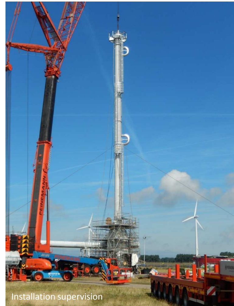
Trial fit Flare tip on riser
