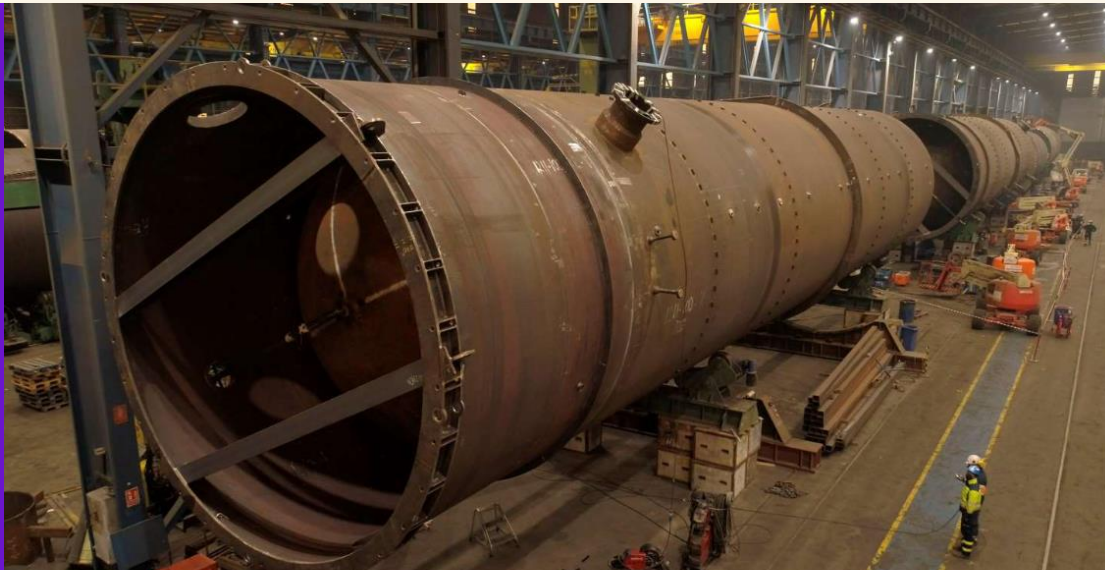
Fabrication of storage tanks by Idesa, Spain
