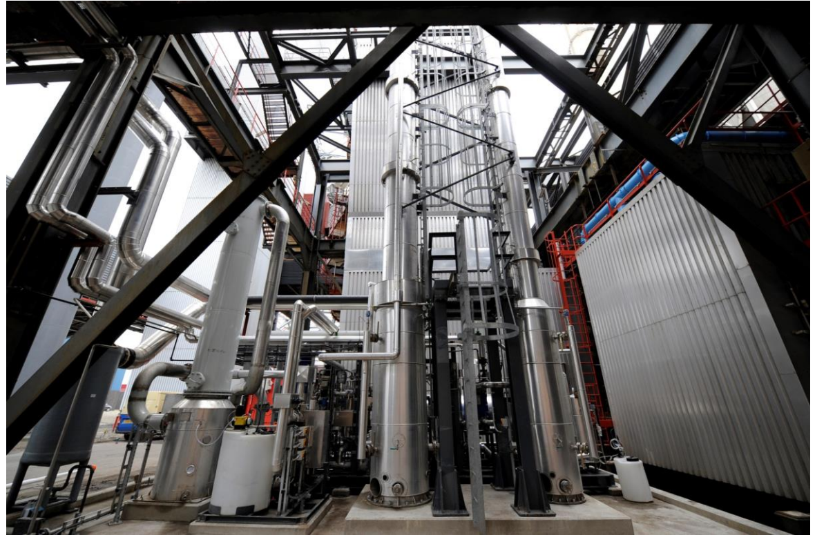
50 cm diameter absorber, capacity 6 ton of CO 2 captured per day
