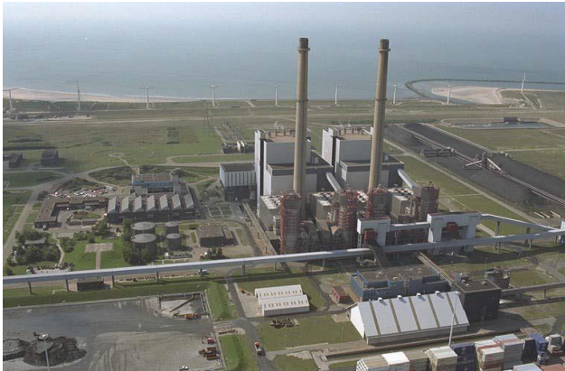
Hard coal fired power plant Maasvlakte, Netherlands
