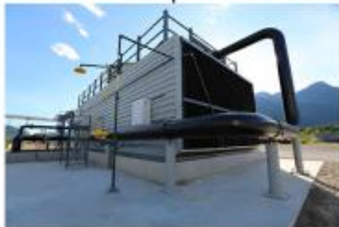
Pilot plant performance data
