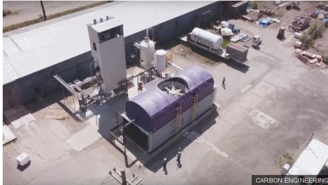
The pilot plant has been built in British Columbia and is extracting about a tonne of CO 2 every day
